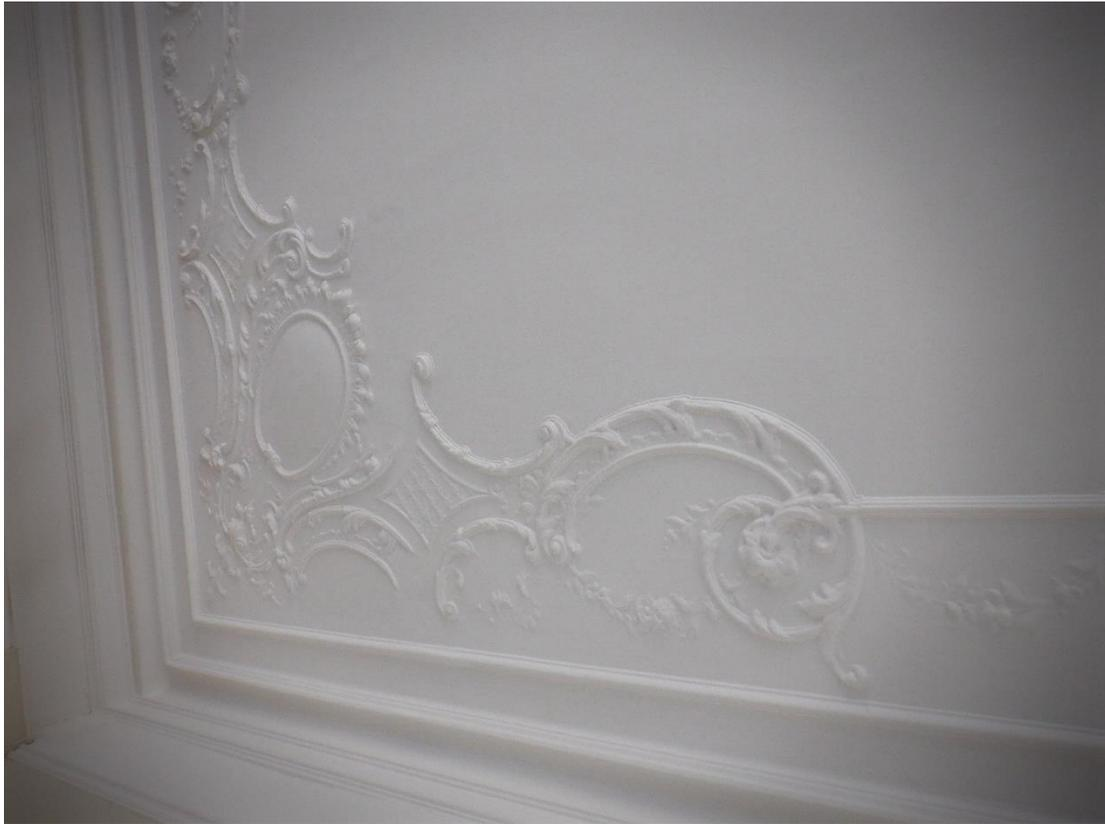
Plate 43. Detail of plaster ceiling mouldings
