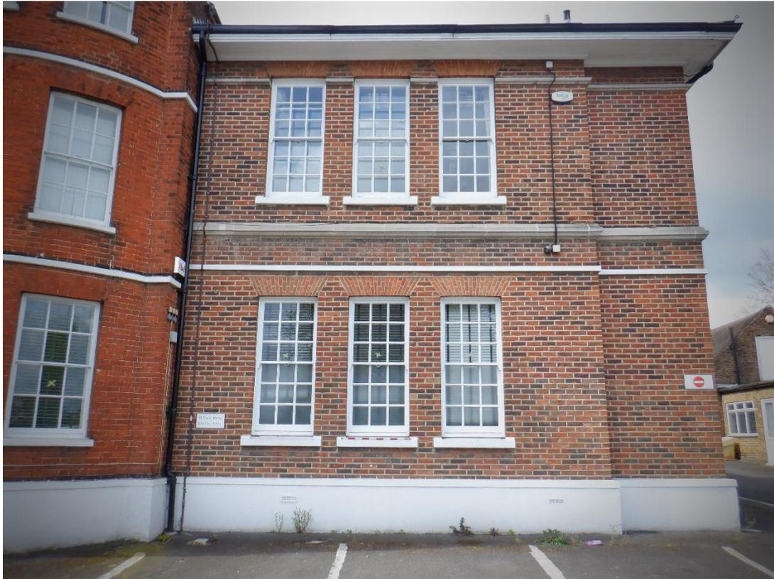
Plate 14. Later build to the right of original building to the left (1m scale)
